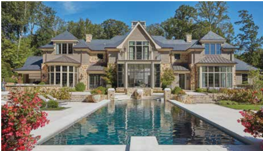
Shingles mingle with stone on the rear façade of a custom Maryland home constructed by Pyramid Builders and designed by Vincent Greene Architects. DAVID BURROUGHS
